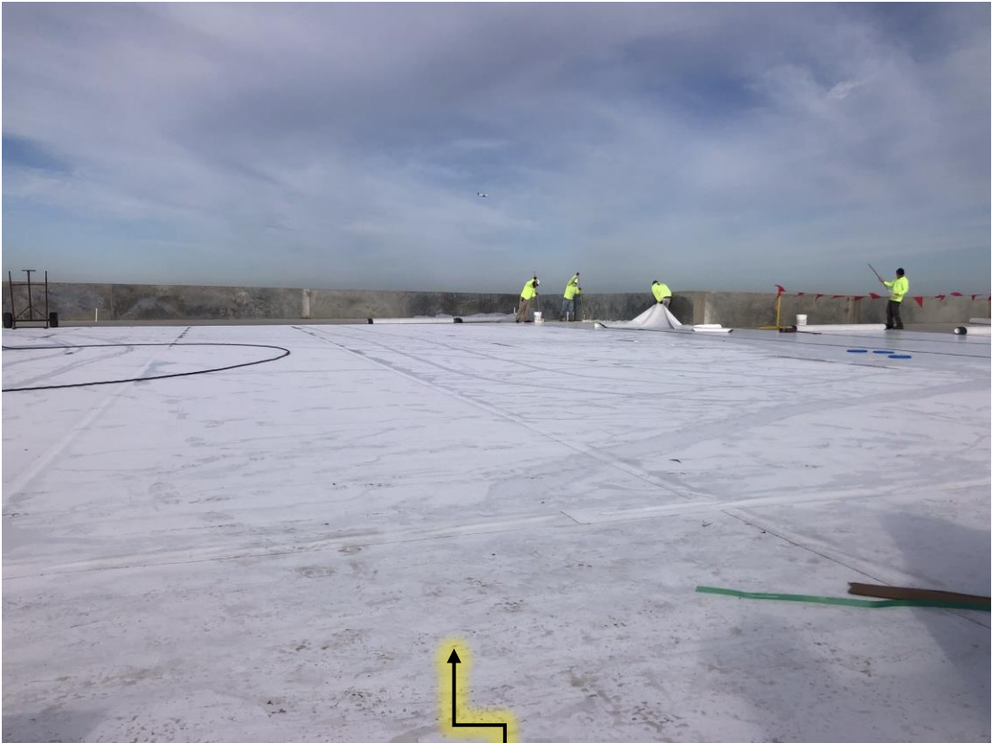
Final Parts of Roofing System Being Installed
