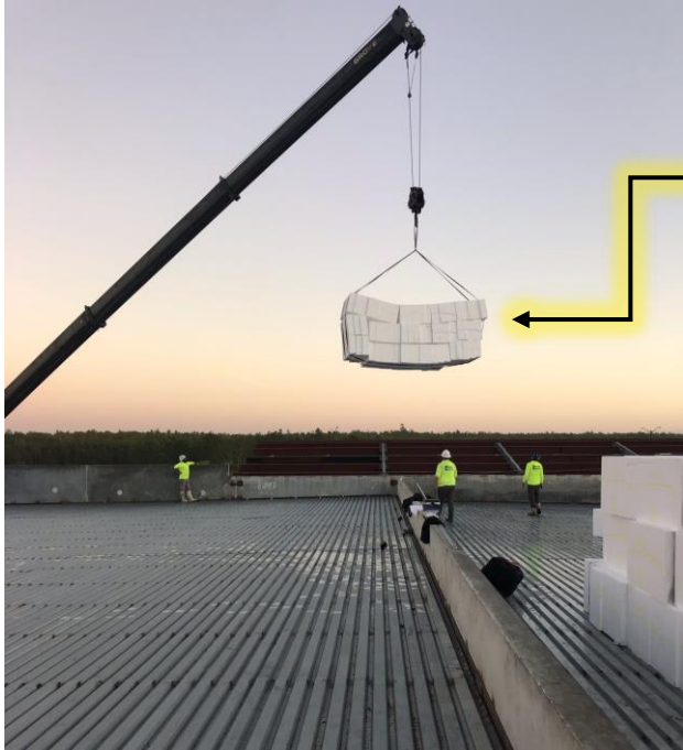
Roofing Material Being Loaded and Installed
