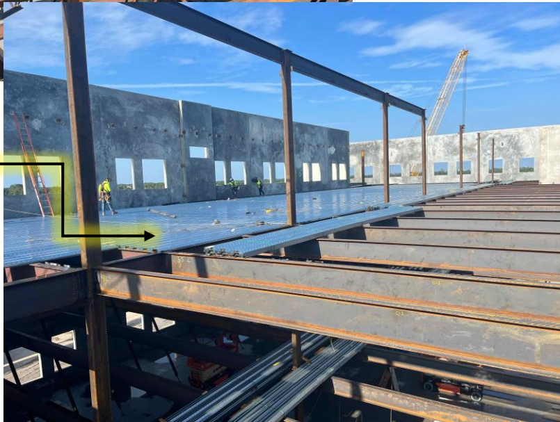
Installing Floor Deck Over Structural Steel
